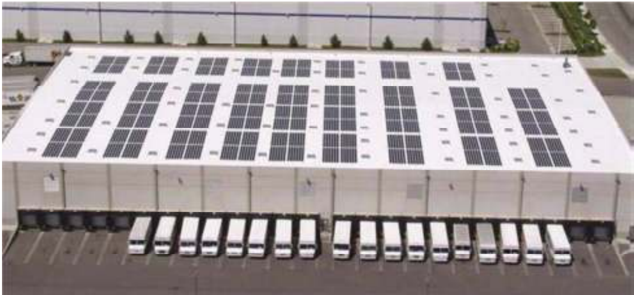
PV integrated roofing at warehouse Frito-Lay Plant, Torrance, CA. Frito-Lay Warehouse
